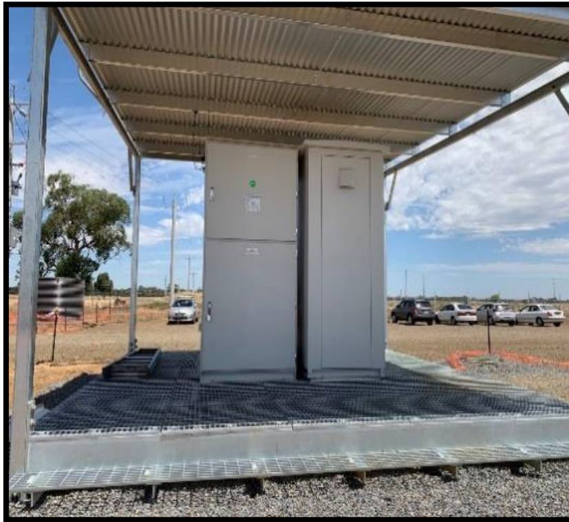
Figure 15 Typical HV switchboard and platform (Source: ACEnergy)
