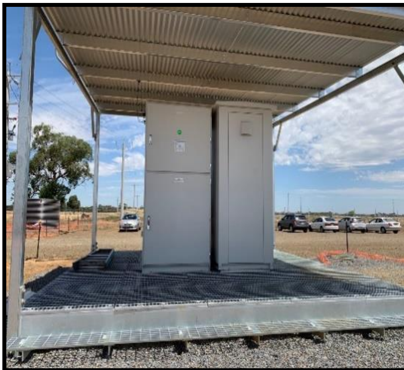
Figure 15 Typical HV switchboard and platform (Source: ACnergy)
