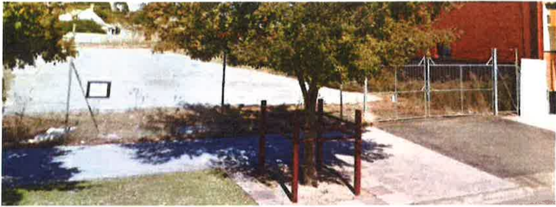
Fig 3: Google "Streetview" showing existing fence – 2.4m high overall with chain mesh and barbed wire Apr 2017
