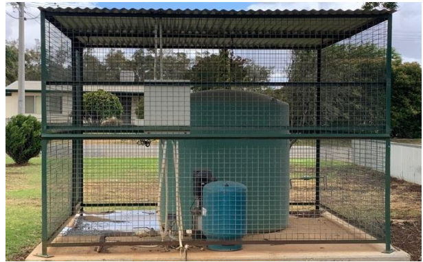
Figure 11 – Water tank enclosure
