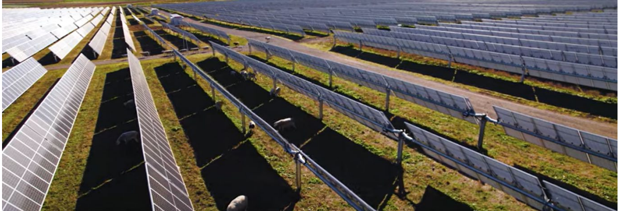
Nextracker SAT system – panels tilted in morning
