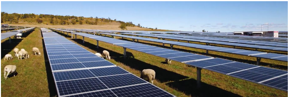
Nextracker SAT system – panels flat at midday
