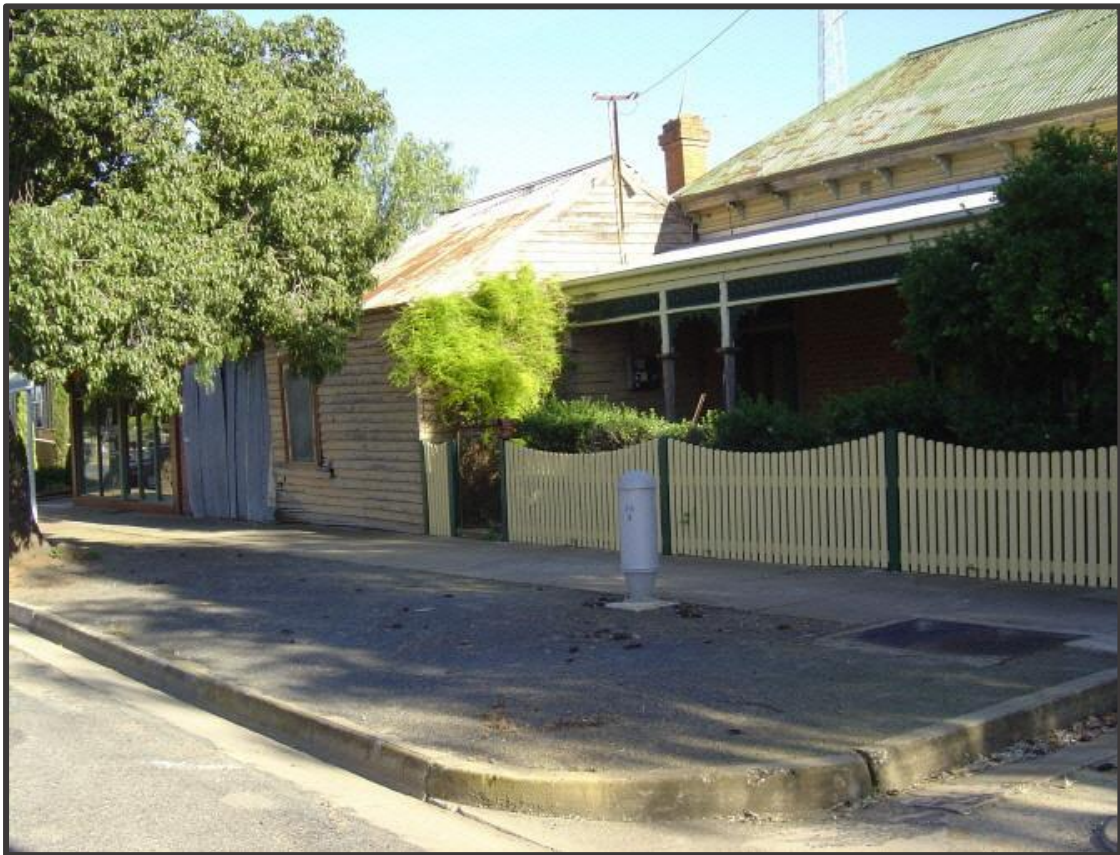
Photograph of the buildings in 2007
