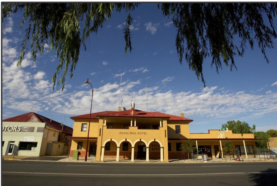
J D Rankin's store was located on the showroom of Jerilderie Motors, to the left of the photograph. H D Harkin's store was located on the hotel driveway and part of the 1928 two storey section. The first two archways of the two storey section are concealing where the Bank of New South Wales was located. The single storey section of the hotel on the right is the renovated original part of the hotel, as are outbuildings located immediately behind the single storey section.
