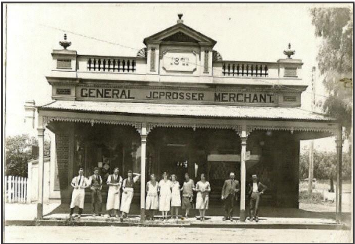
Melbourne House, when leased by J C Prosser (1925-1950) before it was gutted by fire for the second time on Monday, 29 June, 1931. The first fire occurred in March 1892.
