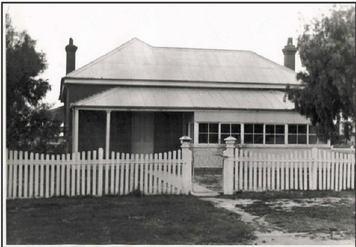
Photograph of Courthouse in 1963, showing section of verandah enclosed.
